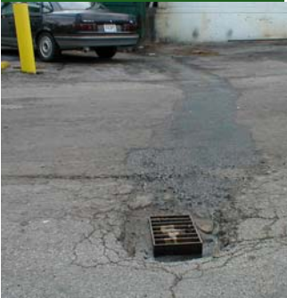
Is your business near a storm drain?
